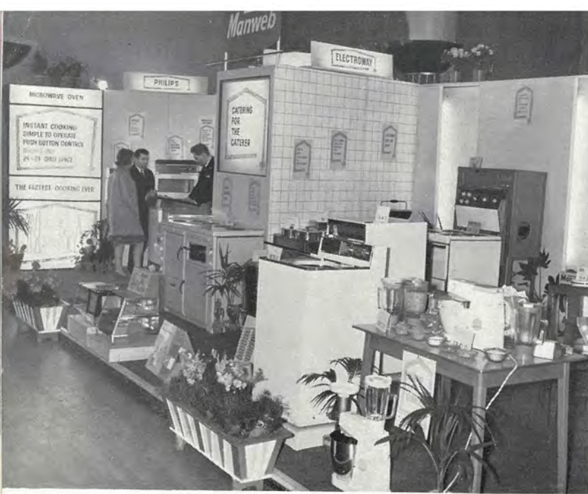
◀ Left: A general view of the electricity stand.
